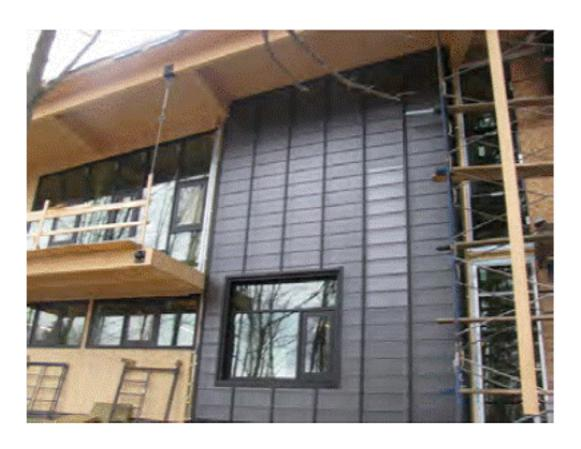
As a first application of its technology, Enerconcept offers the Lubi™ collector, a wall-mounted solar air heater which is entirely made of polycarbonate, deemed so far the best material to withstand impacts from the environment and for wind load resistance. All other parts of the collector, including the structural components and the frames, are made of aluminum.
