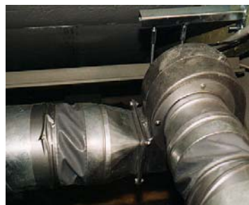
Fig. 3: Flexible duct connections (part of the delivery)
