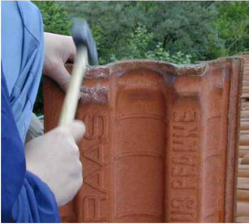
Tap a recess for the roof hook out of the tile
