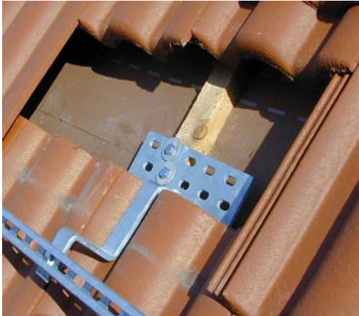
Attached roof hook with screwed-on cross rail
