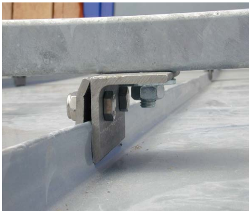
Installation to a standing seam metal roof
