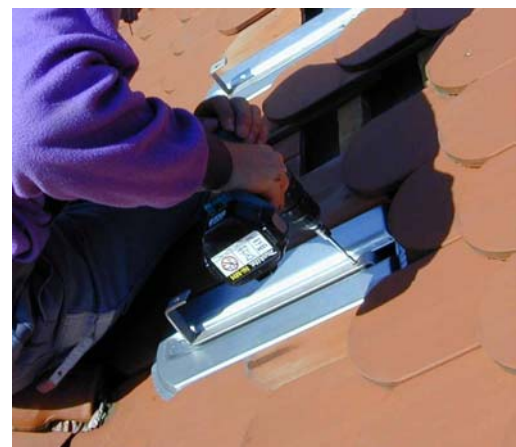
Attachment of a roof hook for slate roofs
